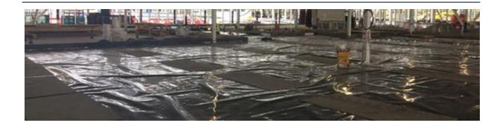
**EPS Evolution VOC** has market leading performance as a Hydrocarbon Barrier and chemical resistant barrier with exceptional resistance to a wide range of pollutants including hydrocarbons, industrial chemicals, toxic waste, natural and radioactive gases; it also acts as a high performance DPM.
